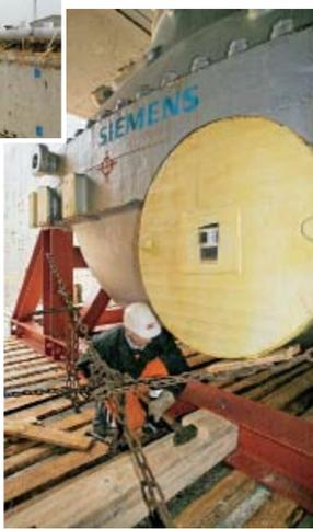
Az Zour's existing gas turbine power plant. Siemens then contracted DB Schenker Global Projects to handle the entire logistics of the project. Approximately 12,200 weight tons - an equivalent of 48,500 freight tons - need to be transported. A single transformer weighs a hefty 392 tons. In Nuremberg an 800-ton crane is used to load the transformer onto a barge for transport to Hamburg, from where it is shipped to Kuwait, and delivered right onto the foundation in Az Zour.
